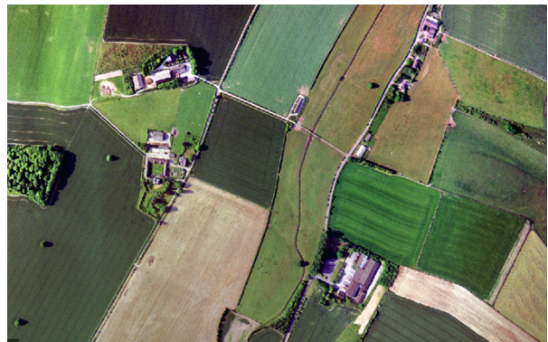
Aerial photograph of site context
