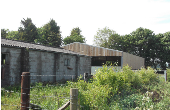
The application site in foreground
